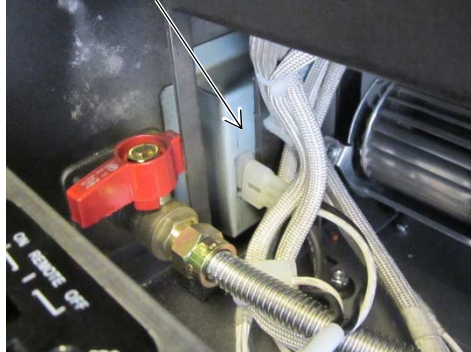
Junction Box (from inside fireplace)
