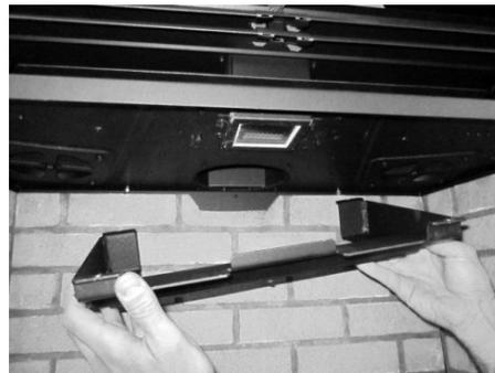
2. Remove the accent light cover plate from the roof of the firebox. Remove the outer 8 screws, not the inner 4 screws.
