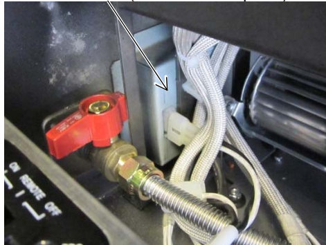
Junction Box (from inside fireplace)
