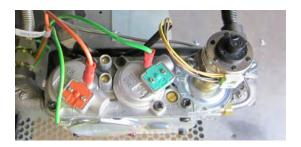
7. Make the gas line connection, bleed the gas line (if applicable), start the heater, and thoroughly leak-test all gas connections and the gas control valve.
